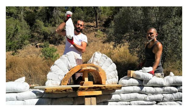
I was kneeling on the wall beside one of the wooden frames, earthbag wedge in hand, while Gürkan fed barbed wire underneath it.
